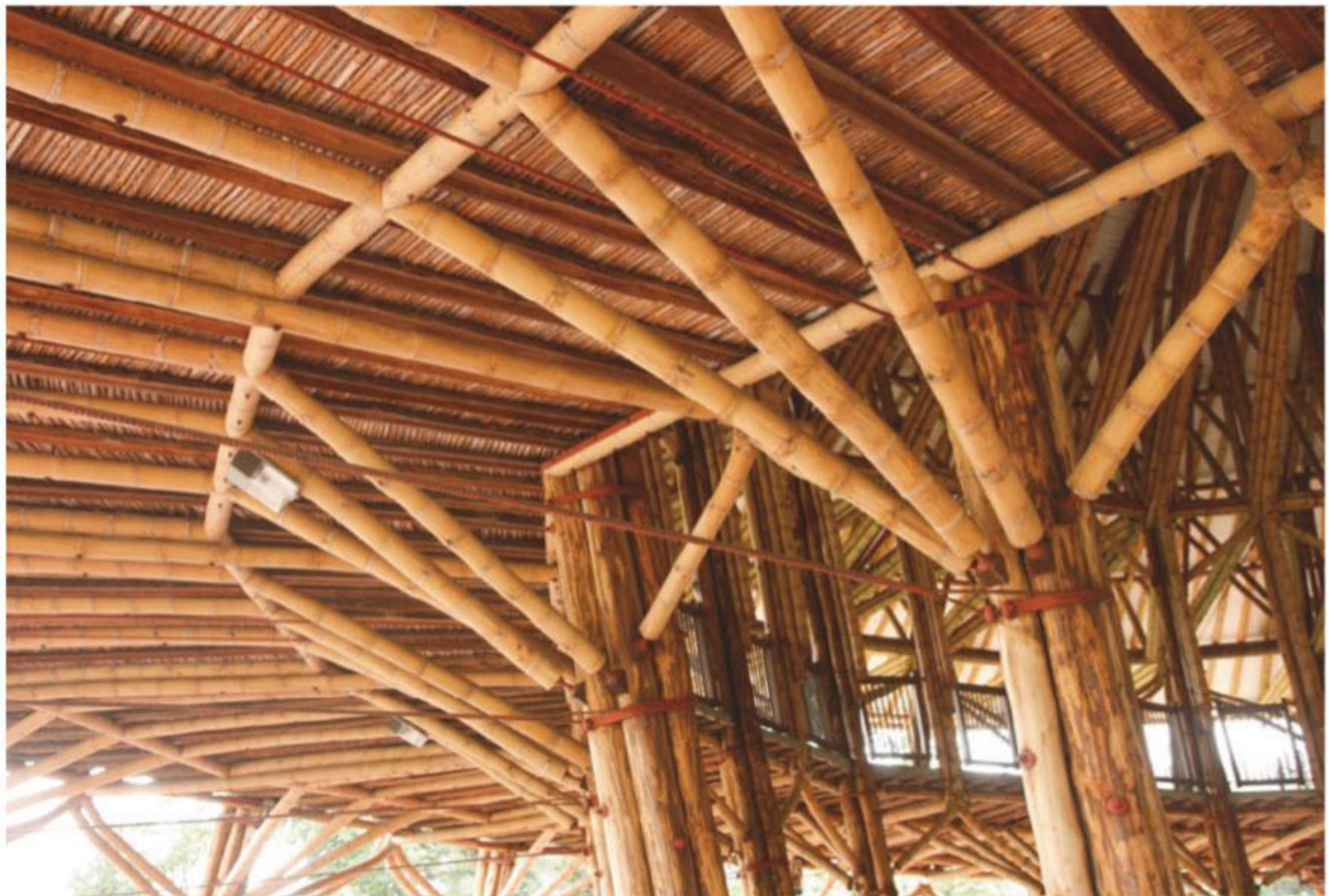
p. 46: Section drawings. p. 47: Detail drawings of the joints. Opposite: Photo of the full-scale prototype taken during construction. This page: Details of the full-scale prototype.
