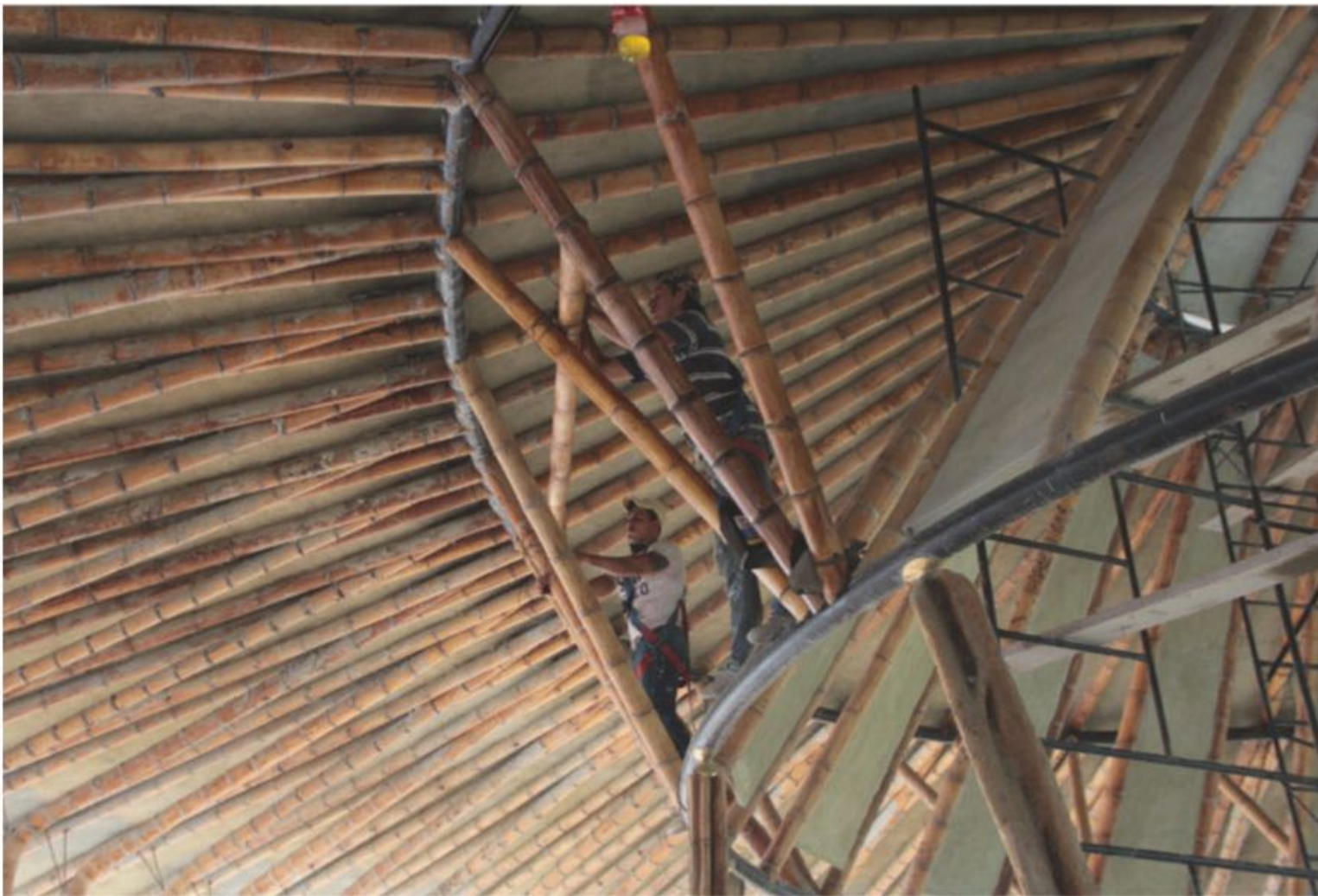
This page, top: Central module during construction. This page, bottom: Close-up view of the roof during construction. Opposite, top: Plan. Opposite, bottom: Roof plan and section.
