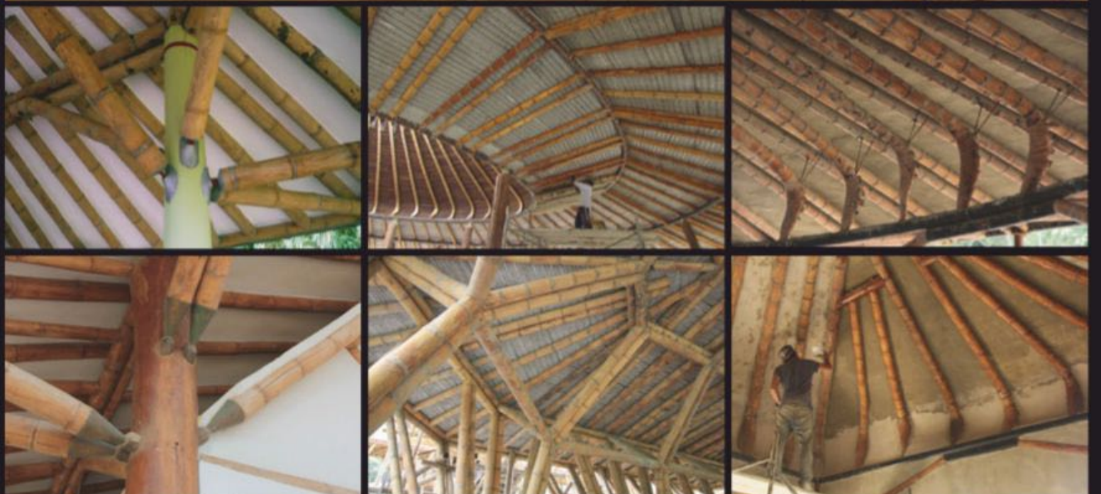
Opposite: Simón Vélez visiting a bamboo forest. This page: Detail of the structure using bamboo or wood. From the top, left to right: Contemplation Pavilion (pp. 192–197), Casa Quindio (pp. 100–105), Casa Aya (pp. 144–153), Tropical House (pp. 154–163), Casa Cartagena (pp. 134–137), Rock Climber's House (pp. 184–191), Tropical House.
