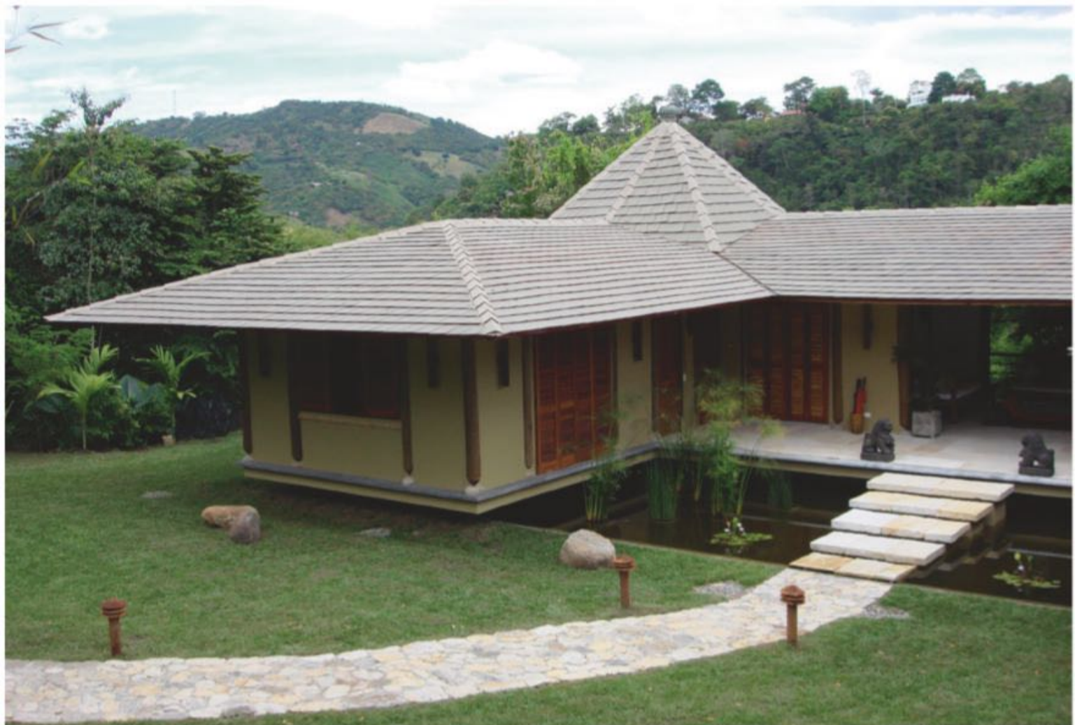
pp. 108–109: Living area sheltered by a large roof. Opposite, top: Long section. Opposite, bottom: Short sections. This page, top: Aerial view of the roof. This page, bottom: View towards the entrance from the approach.
