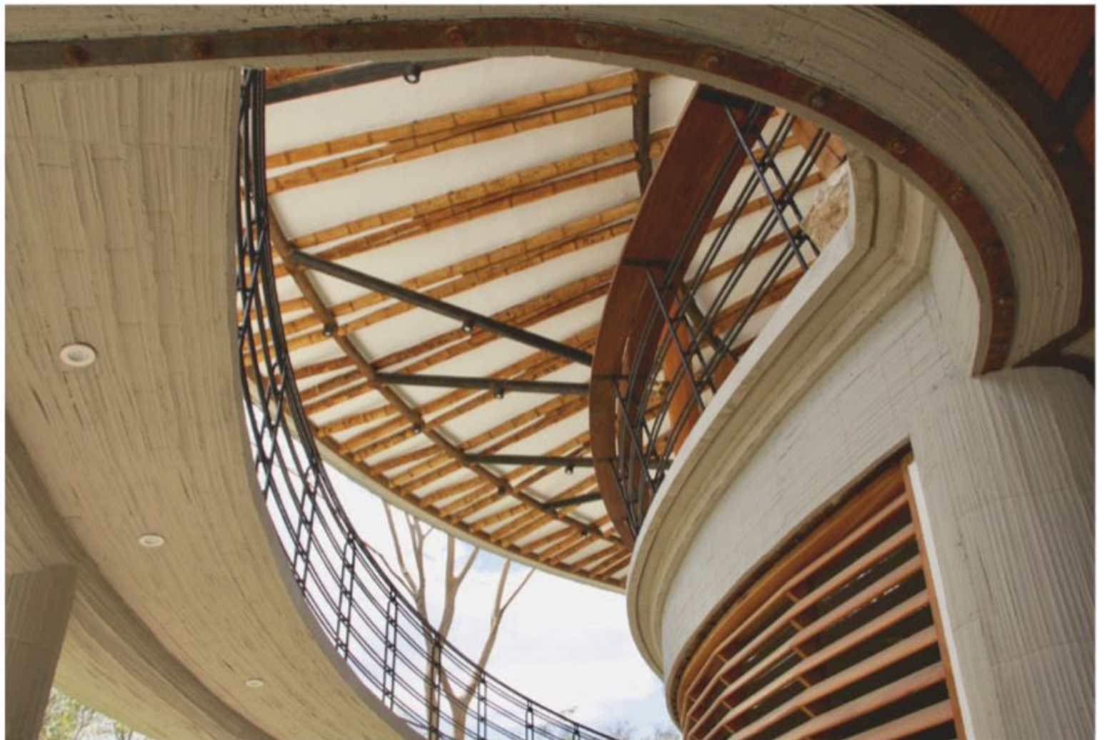
pp. 150-151: Roof of the central module during construction. Opposite, top: Ceiling plan of the central module. Opposite, bottom: Section of the central module. This page, top: Looking up at the roof structure. This page, bottom: View from under the ramp.
